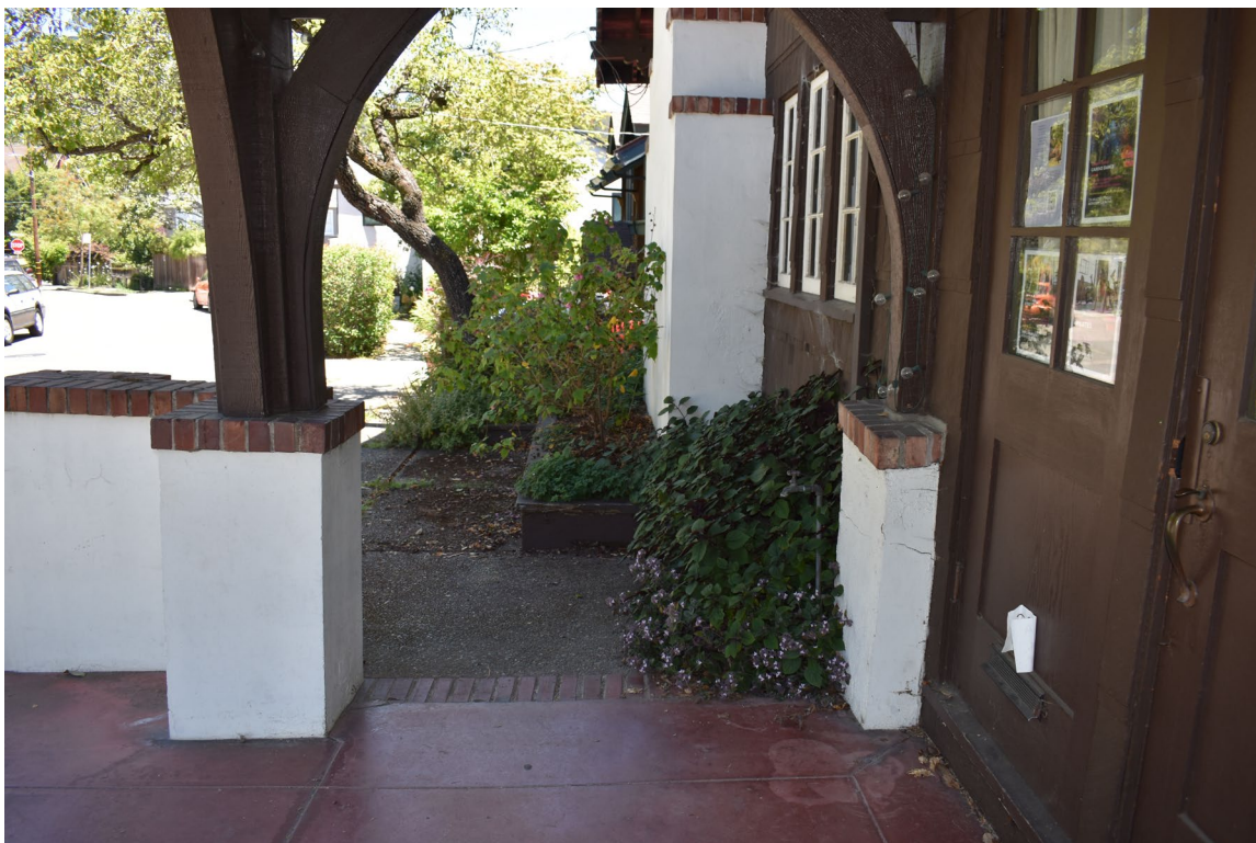
Photo 27. 214 Hillcrest Road - Claremont Club_Berkeley_CA_Photo_0027. SITE VIEW: Planter box along the primary façade, view east.
