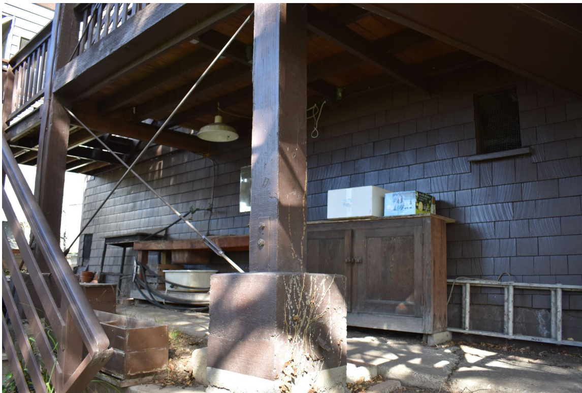
Photo 20. 214 Hillcrest Road - Claremont Club_Berkeley_CA_Photo_0020. SITE VIEW: View of the basement level of the rear south façade, looking northwest.
