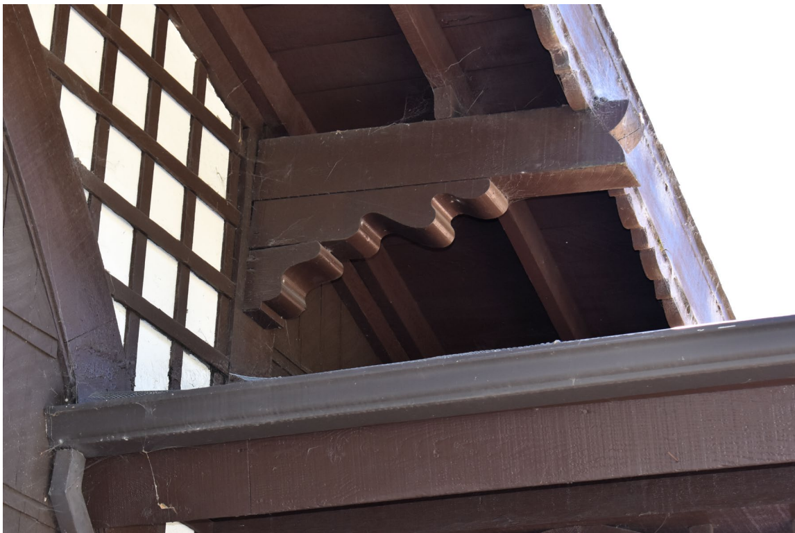
Photo 8. 214 Hillcrest Road - Claremont Club_Berkeley_CA_Photo_0008. SITE VIEW: Detail view to the southwest of spandrels, paneled soffit, and decorative rafters at the primary gable end.
