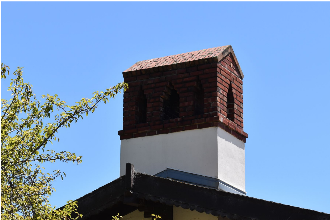
Photo 6. 214 Hillcrest Road - Claremont Club_Berkeley_CA_Photo_0006. SITE VIEW: Detail view southeast of the chimney flue opening.
