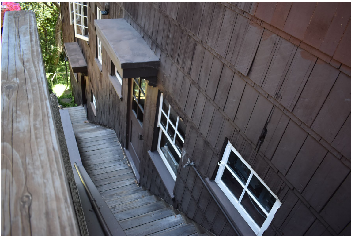
Photo 12. 214 Hillcrest Road - Claremont Club_Berkeley_CA_Photo_0012. SITE VIEW: Oblique view of the lower two floors of the east façade, looking south.
