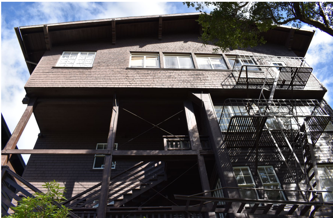
Photo 14. 214 Hillcrest Road - Claremont Club_Berkeley_CA_Photo_0014. SITE VIEW: Rear façade, view north.
