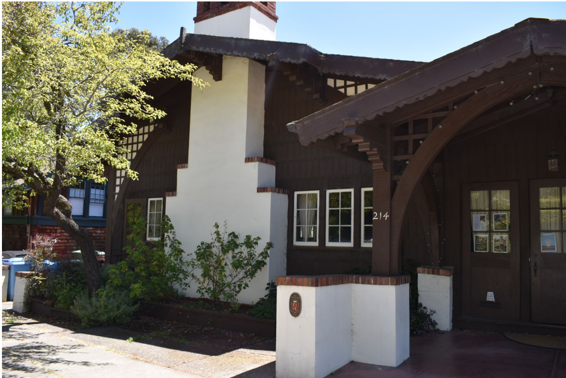
Photo 5. 214 Hillcrest Road - Claremont Club_Berkeley_CA_Photo_0005. SITE VIEW: Oblique view southeast of the central chimney.
