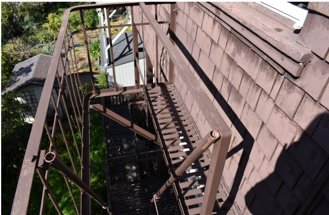
Photo 16. 214 Hillcrest Road - Claremont Club_Berkeley_CA_Photo_0016. SITE VIEW: Oblique view of the fire escape accessed from the upper floor of the rear façade, view west.
