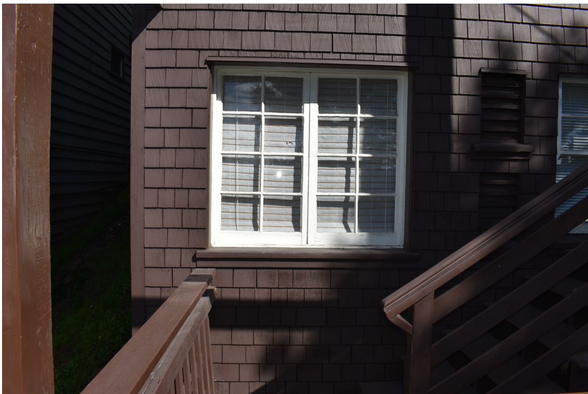
Photo 17. 214 Hillcrest Road - Claremont Club_Berkeley_CA_Photo_0017. SITE VIEW: View of the (residential) third floor on the rear south façade, looking north.
