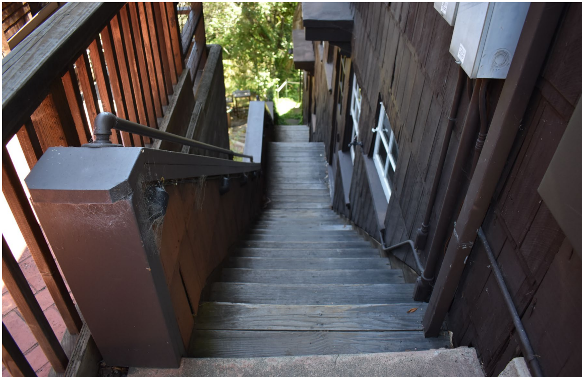
Photo 28. 214 Hillcrest Road - Claremont Club_Berkeley_CA_Photo_0028. SITE VIEW: Wood-frame staircase along the eastern façade, view south.
