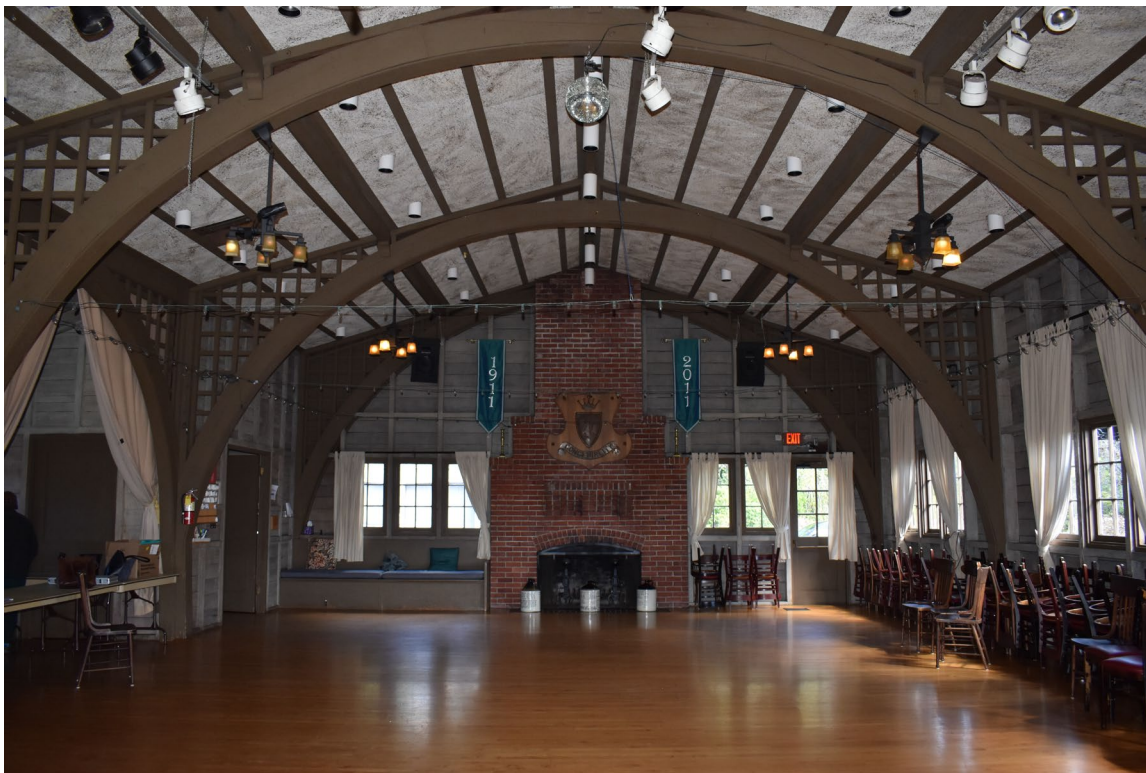
Photo 24. 214 Hillcrest Road - Claremont Club_Berkeley_CA_Photo_0024. SITE VIEW: Interior view of the main meeting hall space, looking north.
