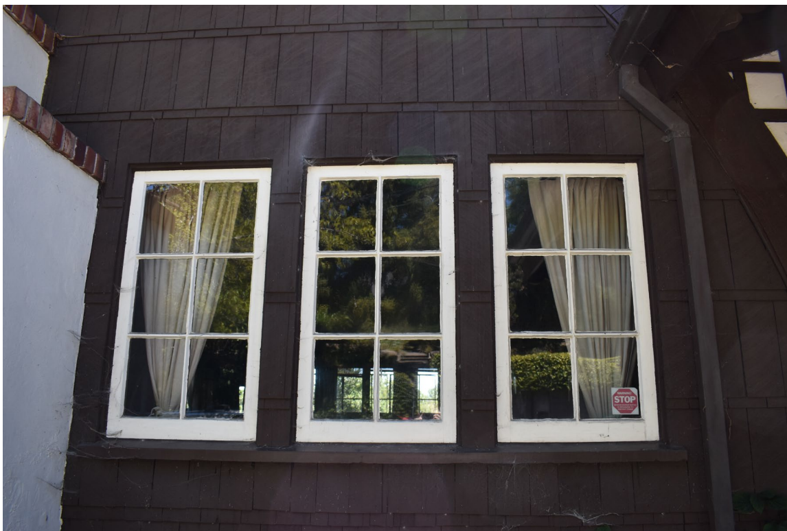
Photo 7. 214 Hillcrest Road - Claremont Club_Berkeley_CA_Photo_0007. SITE VIEW: Detail view south of wood sash casement windows on the primary façade.
