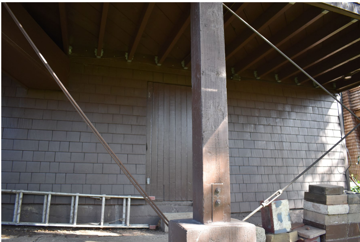
Photo 19. 214 Hillcrest Road - Claremont Club_Berkeley_CA_Photo_0019. SITE VIEW: View of the basement level of the rear south façade, looking north
