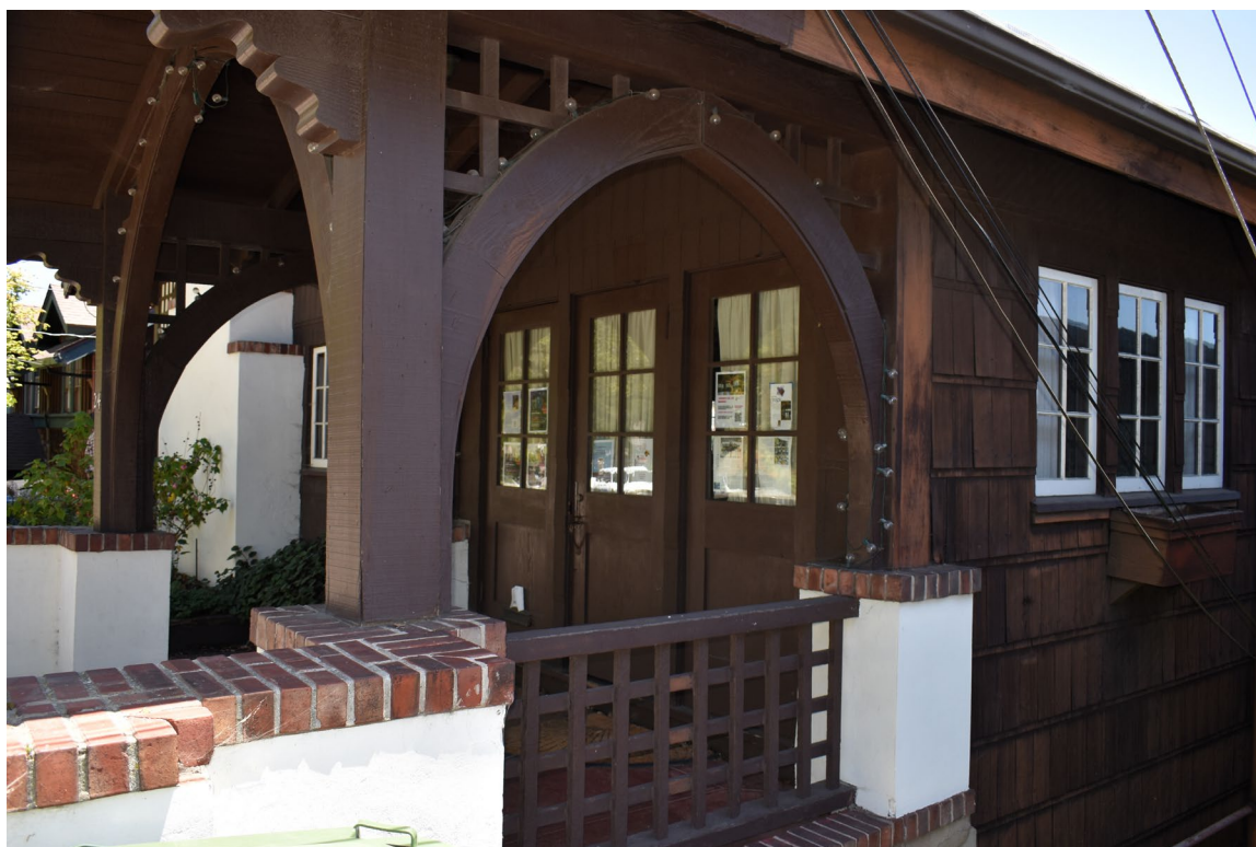
Photo 4. 214 Hillcrest Road - Claremont Club_Berkeley_CA_Photo_0004. SITE VIEW: Oblique view to the southeast of lattice spandrels and banister along the entry portico.
